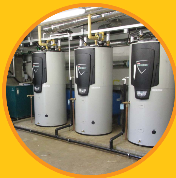
New hot water heaters at Central Village
